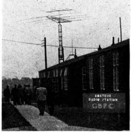
The new rotary beam arrays at G8FC—Headquarters Station, R.A.F.A.R.S.
